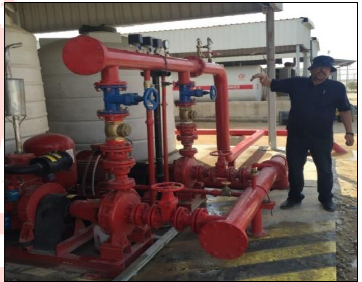
Supply and Installation Firefighting Pump for EMC
