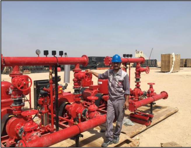
Supply and Installation Firefighting Pump for KPS
